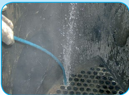
Heat exchanger cleaning – 33 lpm / 800 bar
