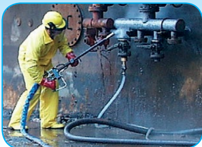
Surface preparation of valve manifold
