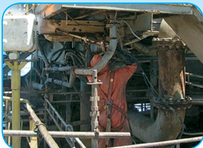
Offshore surface preparation aboard a jack up
