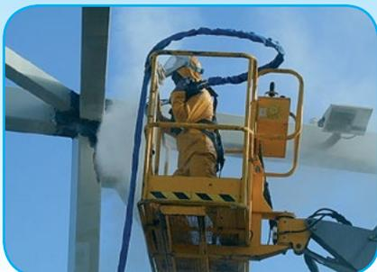
Coatings removal for weld inspection
