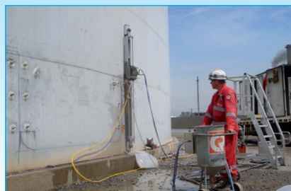
Cutting a section from an oil storage tank
