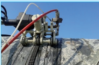
Cutting large a diameter pipe
