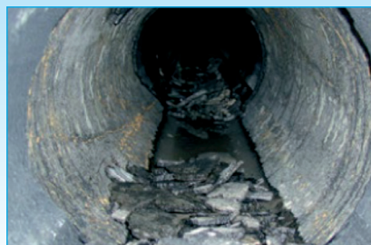
Descaling large diameter pipe, 200lpm at 1000bar
