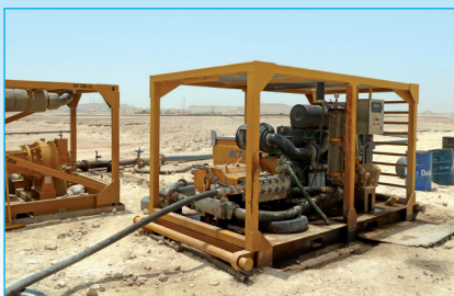
HPS5000DC unit on a pipeline testing project
