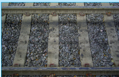
Leaf mulch deposits on rail head before jetting
