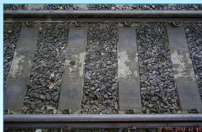
Rail head after cleaning, 200lpm at 500bar
