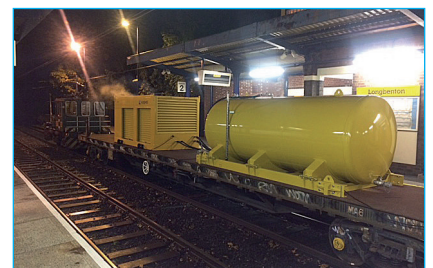
Nexus unit cleaning rail heads at 83lpm at 1000bar
