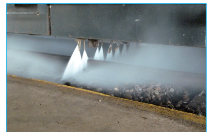
TRTC unit cleaning sleepers at 320lpm at 210bar
